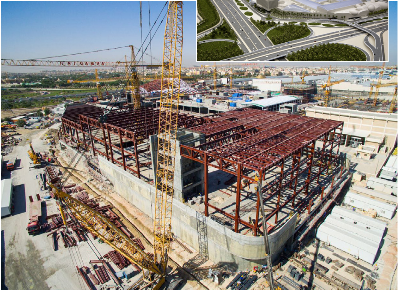
Cinema Steel Structure and Shops
