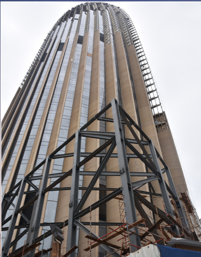
Secondary Steel Works for Façade
